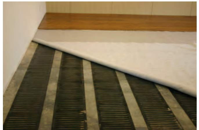
Elements on Concrete, Under Sound Barrier and Bamboo
