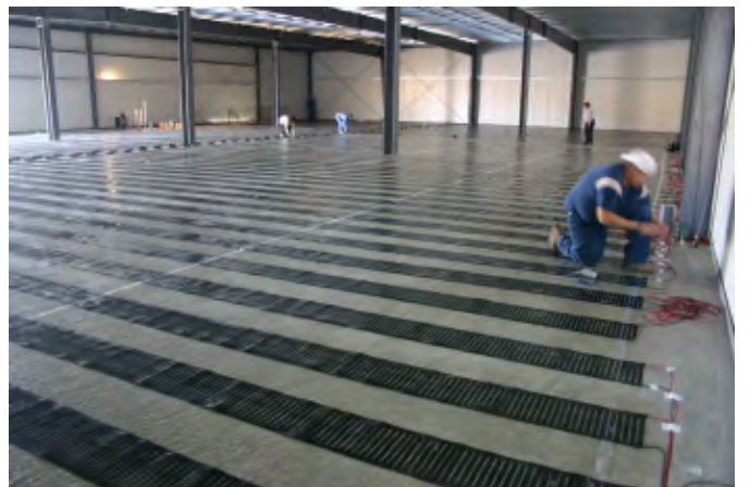
Heating Elements Between Two Layers of Concrete
