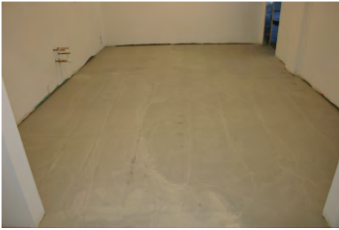
Element Covered by Floor Leveler
