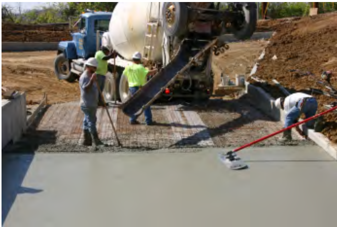
STEP Snowmelt in Vinyl Under Concrete
