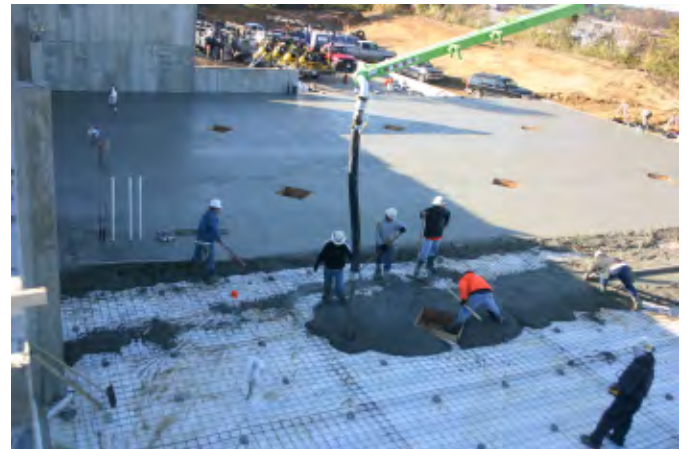
Heating Elements over Insulation and Under 6" Slab
