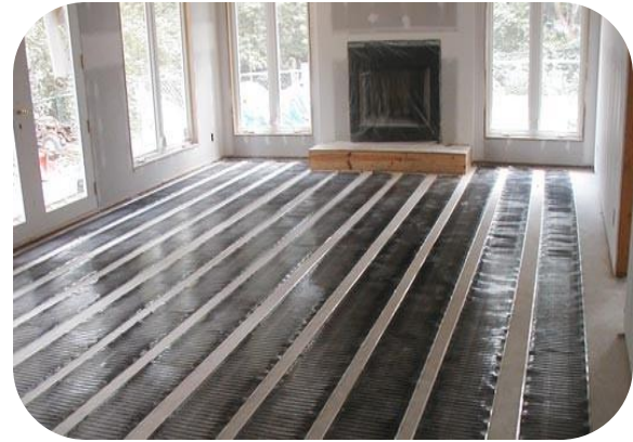
Radiant heating systems, like STEP Warmfloor (pictured above), provide heat from the floor up.
